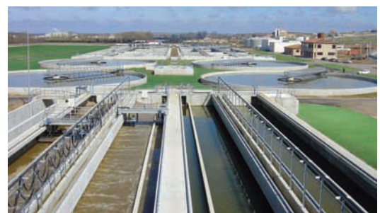
Wastewater treatment plant in Salamanca.
