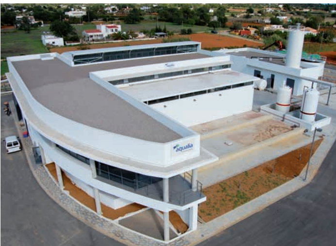
Desalination plant in Santa Eulalia (Ibiza).
